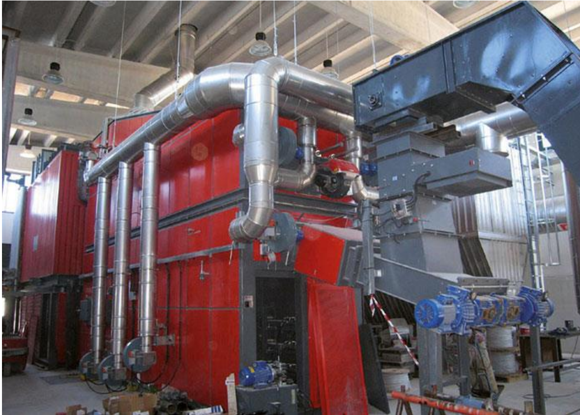
Figure 18 Uniconfort boiler installed at Fiusis power plant (Italy) that fires olive trees prunings for CHP production.
