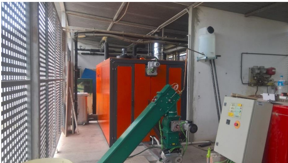
Figure 16: Heating of a swimming pool in Calpe (Spain) with pruning residues. Boiler model: RHK AK300 from Heizomat.
